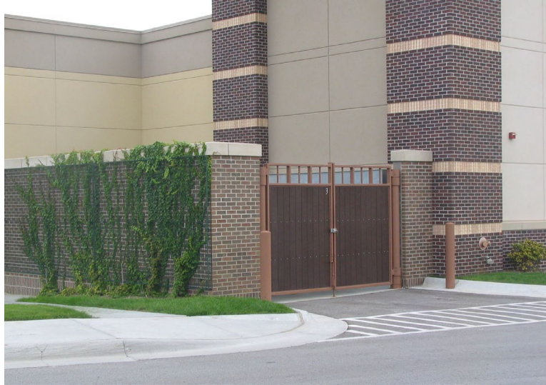
Photo 9—Typical Trash/Service area screen
