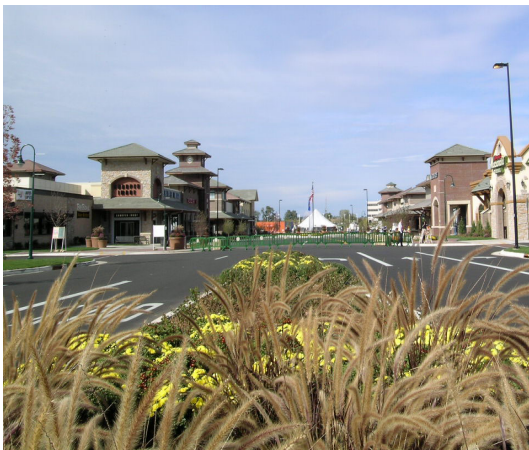
Photo 17—Perimeter landscaping at parking area
