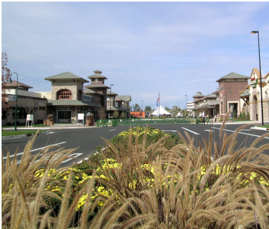
Photo 17—Perimeter landscaping at parking area
